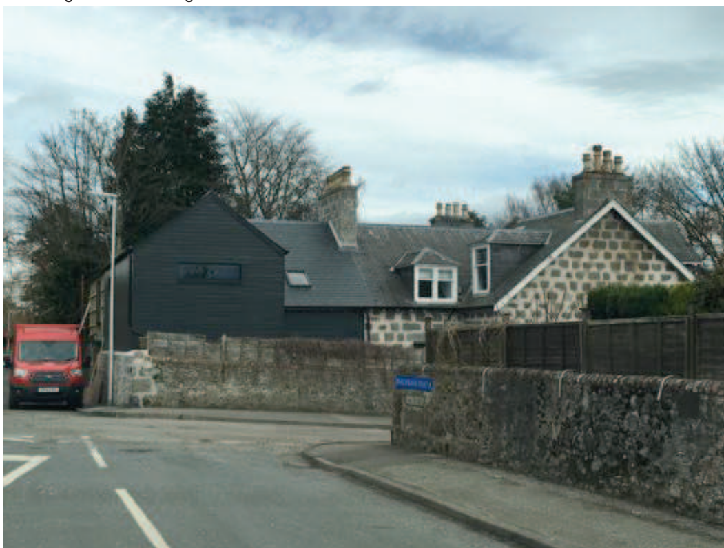
Fig 02 Unconditionally Approved Extension at Junction between Marchbank Road and Golf Road. The extension is built onto the rear and adjoining neighbours boundary. The extension forms a non-traditional courtyard and has an eaves height, in part, that is higher than the original house . P121792
