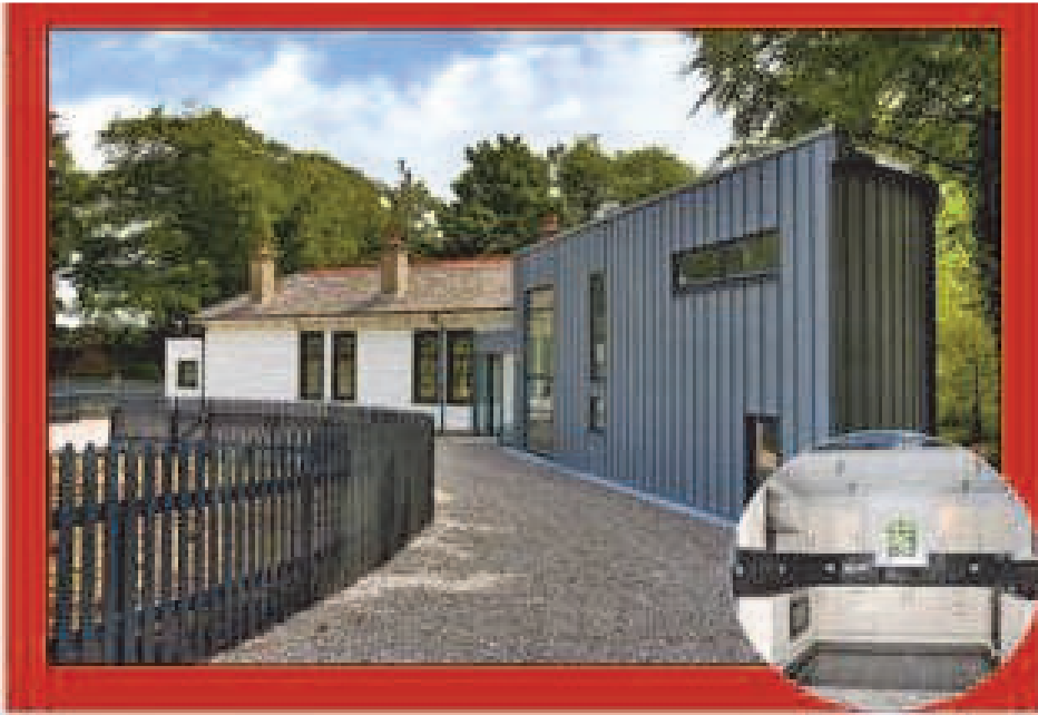
Fig 01 Use of Zinc Cladding to extend the Former Pittfodels Station. It forms a substantial proportion of the building envelope and enhances the historical building. ,
